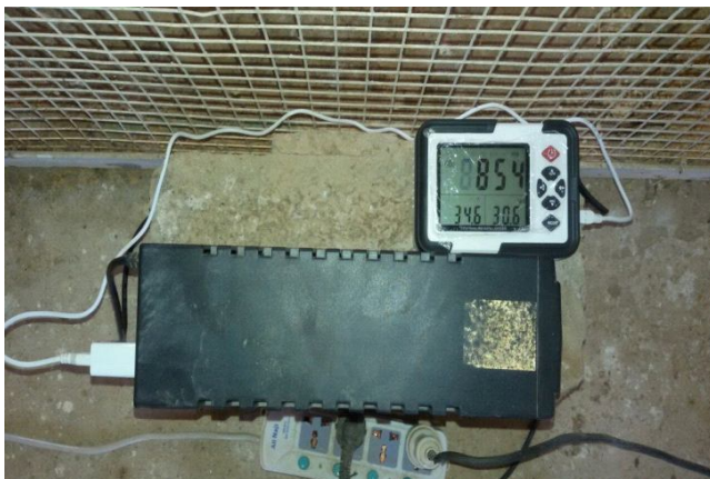
Picture 3: Sensor used to measure carbon dioxide, temperature, relative humidity and dew point.
